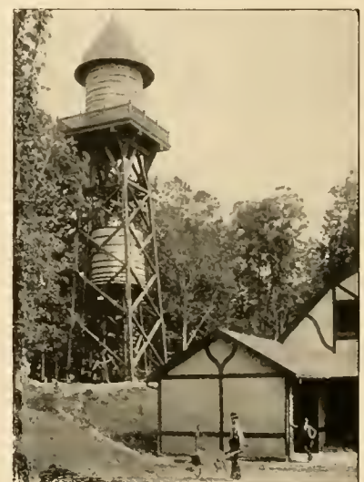
Corcoran Water Tower, Roslyn L. I.
